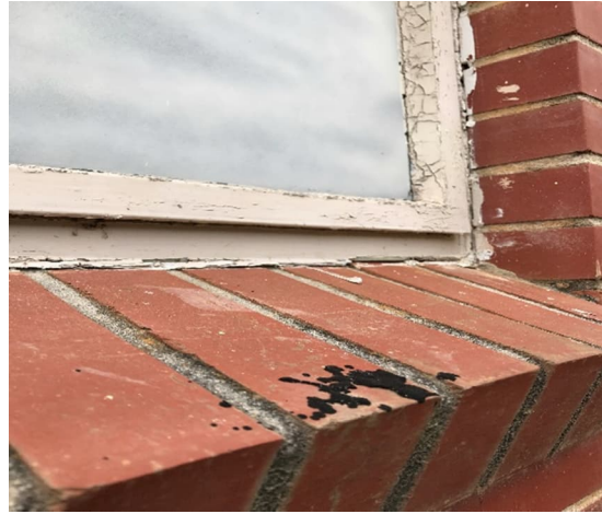
Photo #2 HA# F 8 – Exterior Window Frame Caulk
