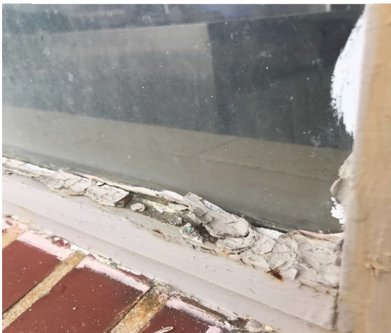
Photo #5 HA# E 16 – Exterior Window Glazing HA# E 17 – Exterior Window Frame Caulk
