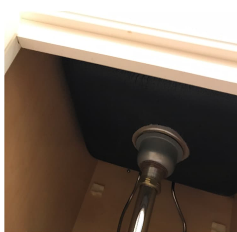
Photo #4 HA# D 9 – Black Sink Coating
