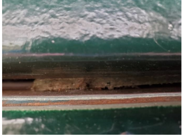
Photo #6 HA# D 11 – Heating Cabinet Liner Panels
