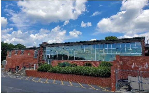
Photo #1 Building E Exterior
