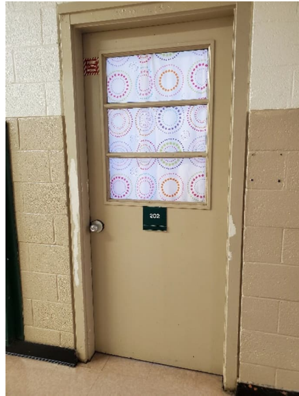
Photo #8 HA# A 26 – Fire Doors (multiple types)
