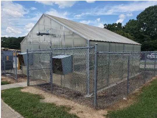
Photo #1 Greenhouse Exterior
