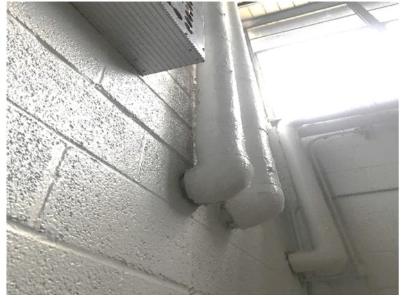
Photo #2 HA# G 2 – 4" Canvas Pipe Elbow Insulation Hot Water (Old Gym)
