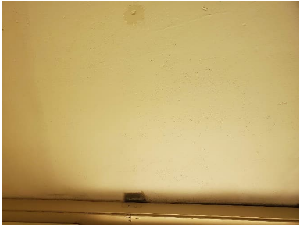
Photo #5 HA# D 10 – Acoustical Plaster Ceilings
