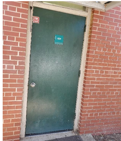
Photo #6 HA# F 14 – Fire Doors (multiple types)
