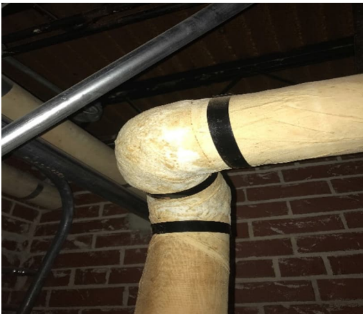
Photo #3 # A 15 – 1" Pipe Elbow Insulation
