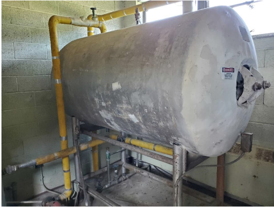
Photo #7 HA# G 9 – Tank Insulation (Old Gym)
