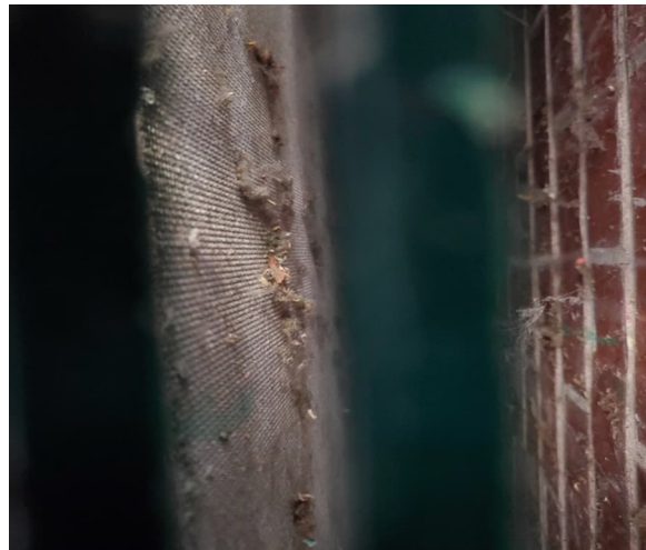
Photo #6 HA# C 10 – Heating Cabinet Liner Panels
