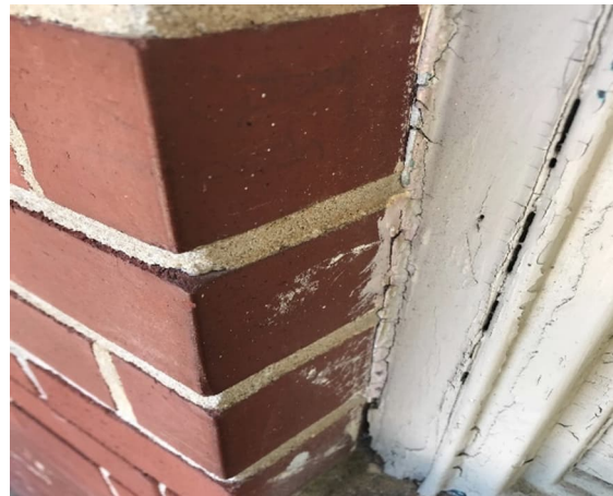
Photo #4 HA# C 8 – Exterior Window Caulk
