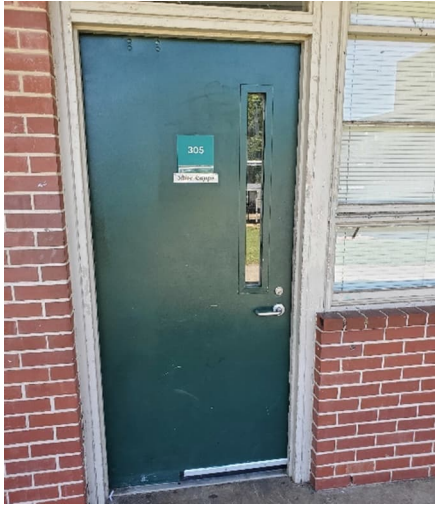
Photo #7 HA# C 11 – Fire Doors (multiple types)
