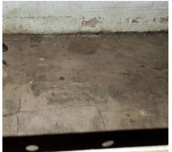
Photo #6 HA# G 8 – 9"x9" Floor Tile and Mastic (Old Gym)
