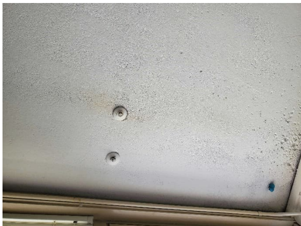
Photo #5 HA# C 9 – Acoustical Plaster Ceilings
