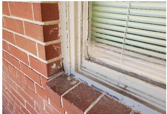
Photo #2 HA# D 6 – Exterior Window Caulk HA# D 7 – Exterior Window Glazing
