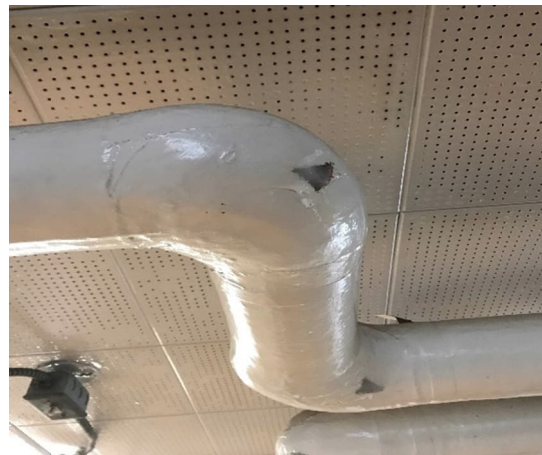
Photo #4 HA# E 11 – 2" Pipe Elbow Insulation
