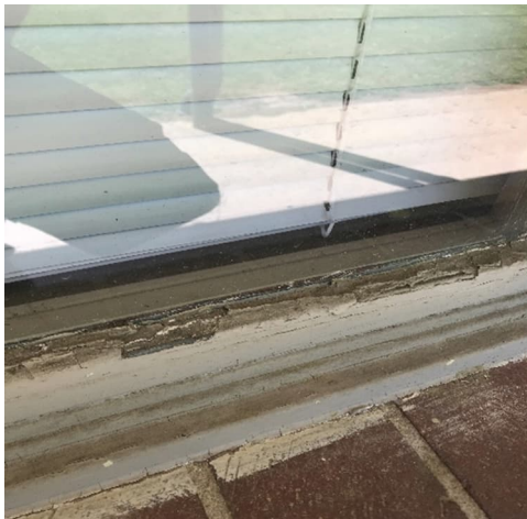
Photo #3 HA# C 7 – Exterior Window Glazing
