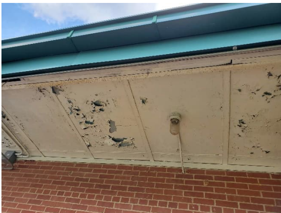
Photo #5 HA# F 13 – Cementitious Panels
