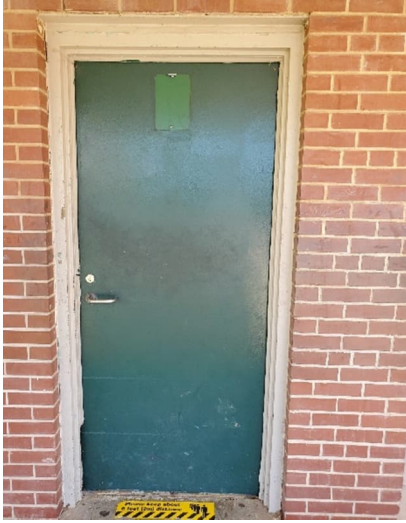
Photo #5 HA# H 10 – Fire Doors (multiple types)
