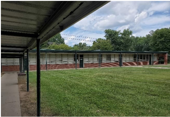
Photo #1 Building H Exterior
