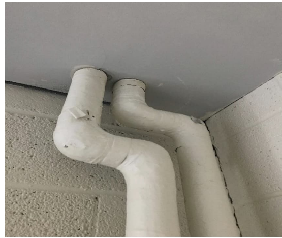
Photo #2 HA# B 3 – 1" Pipe Elbow Insulation
