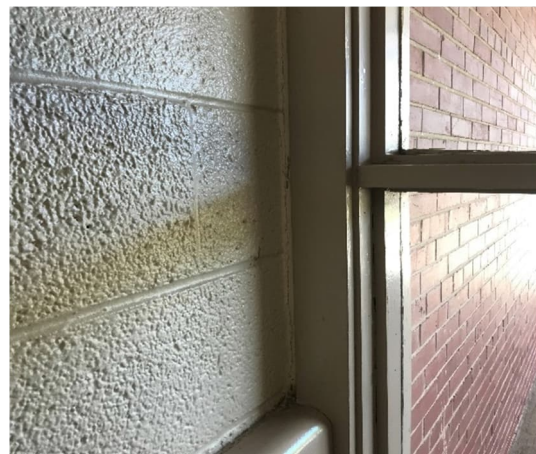
Photo #4 HA# B 16 – Interior Window Caulk
