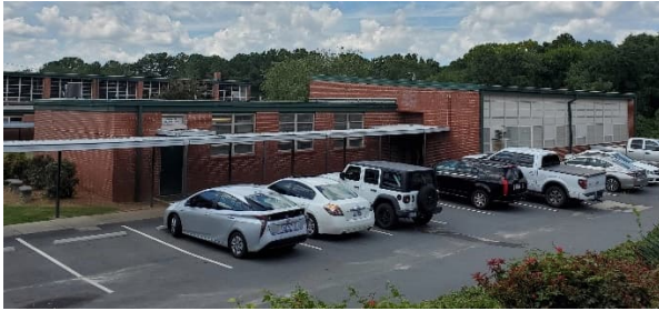
Photo #1 Building F Exterior
