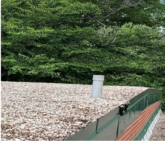
Photo #7 HA# FR 3 – Silver Paint Penetrations
