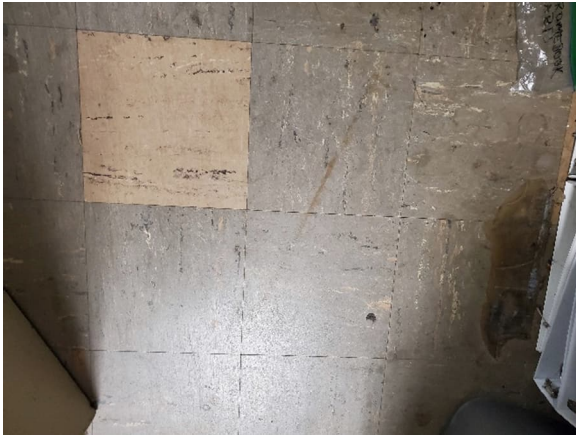
Photo #7 HA# B 24 – 9"x9" Grey Floor Tile & Mastic HA# B 25 – 9"x9" Tan Floor Tile & Mastic
