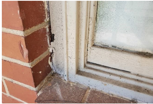
Photo #2 HA# H 6 – Exterior Window Glazing HA# H 7 – Exterior Window Frame Caulk
