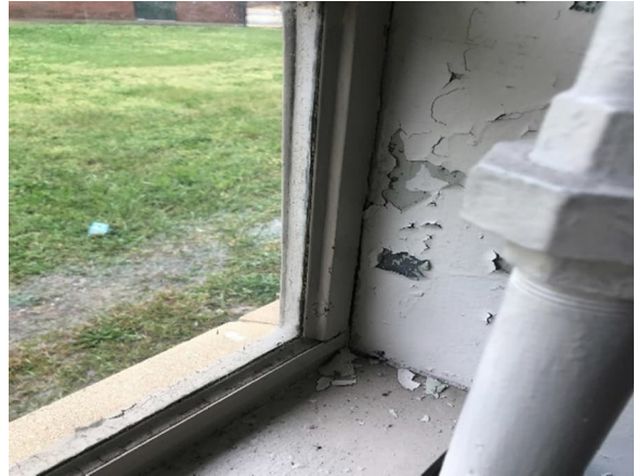
Photo #2 HA# A 6 – Interior Window Caulk
