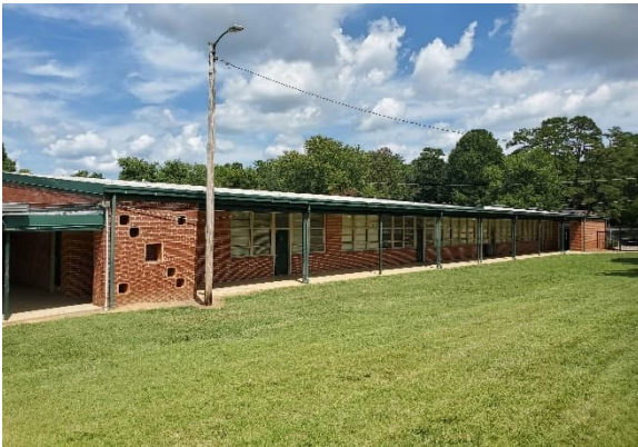
Photo #1 Building D Exterior
