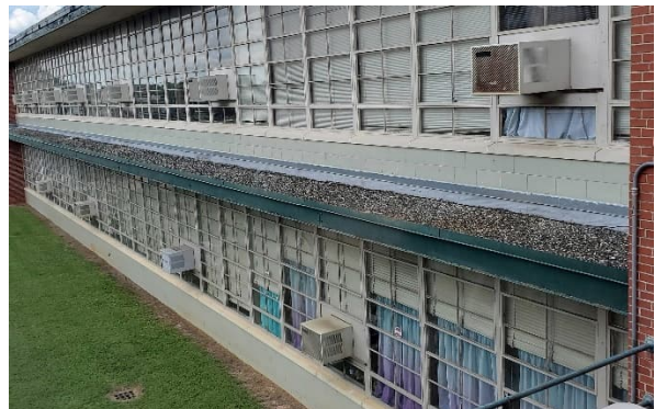
Photo #10 HA# AR 9 – Roof Flashing HA# AR 10 – Gray Roof Caulk
