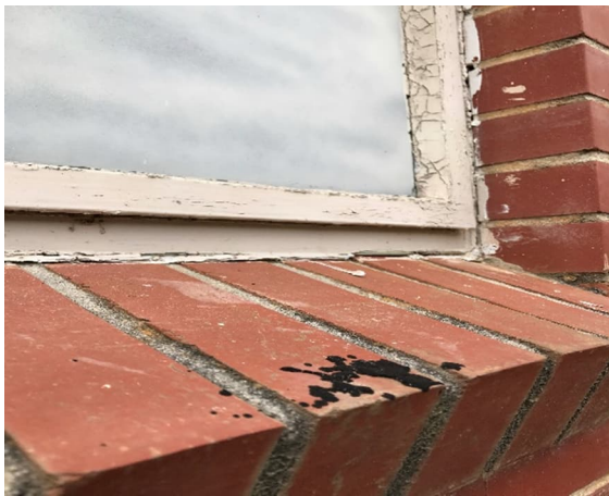
Photo #3 HA# G 4 – Exterior Window Frame Caulk (Old Gym)
