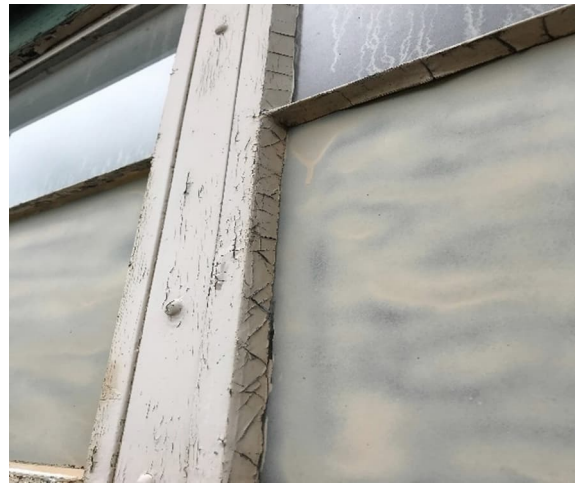
Photo #4 HA# G 5 – Exterior Window Glazing (Old Gym)
