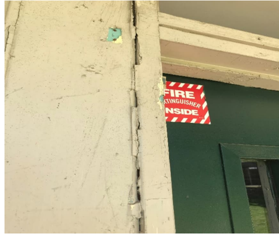
Photo #2 HA# C 6 – Exterior Door Caulk
