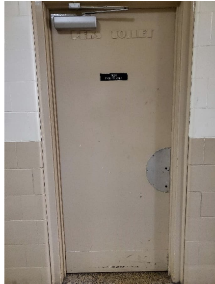
Photo #8 HA# B 26 – Fire Doors (multiple types)
