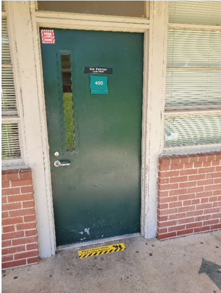
Photo #7 HA# D 12 – Fire Doors (multiple types)
