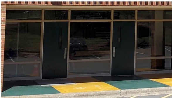
Photo #3 HA# I 21 – Fire Doors (multiple types)
