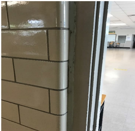
Photo #3 HA# E 10 – Interior Door Caulk
