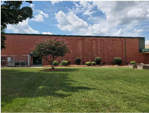
Photo #1 Building B Exterior
