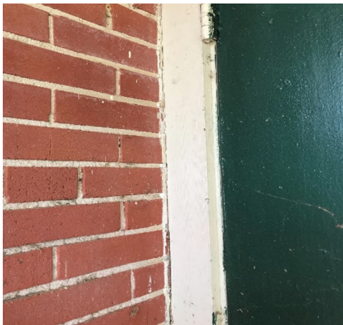
Photo #3 HA# F 9 – Exterior Door Caulk
