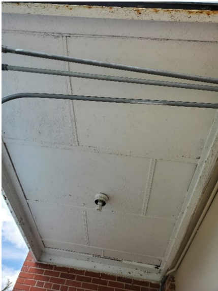
Photo #9 # A 27 – Cementitious Panels
