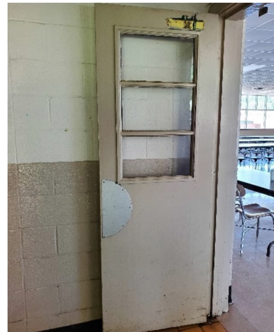
Photo #6 HA# E 25 – Fire Doors (multiple types)
