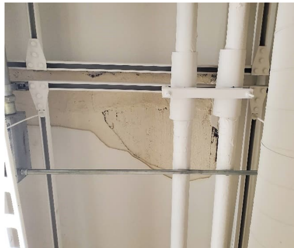
Photo #6 HA# A 24 – Acoustical Plaster Ceilings
