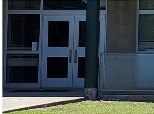
Photo #2 HA# MC 12 – Fire Doors (multiple types)
