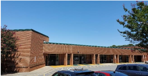
Photo #1 Building I Exterior
