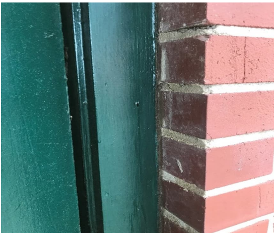
Photo #3 HA# D 8 – Exterior Door Caulk
