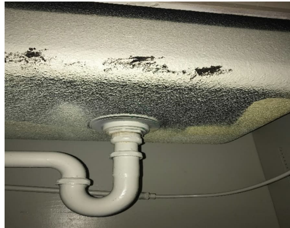
Photo #4 HA# A 17 – White Sink Mastic
